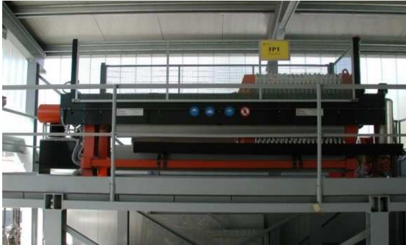
Automatic filter press 800 x 800
